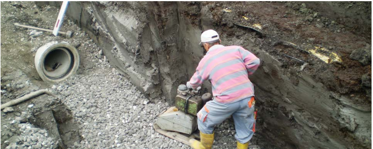
© Foto's: riolering Lustenau, Wilhelm + Mayer © SCHLUSSELBAUER Geomaterials
